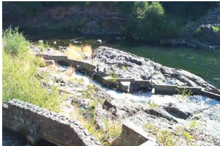
(a) Vertical slot Potter Valley fish ladder on the Eel River in California.
