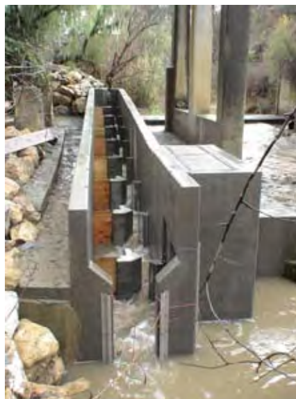
(c) Hybrid vertical slot/pool-and-weir fish ladder on El Jaro Creek, CA.
