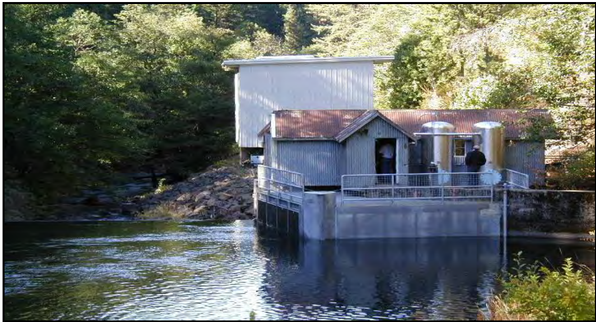
Figure 4-11 Vertical Flat-Plate Fish Screen in Operation
