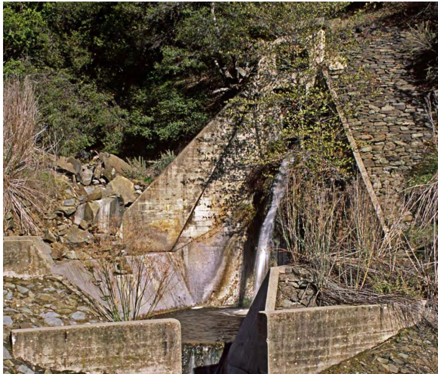
Figure 2-5 Outlet of the Alameda Creek Diversion Tunnel at Calaveras Reservoir
