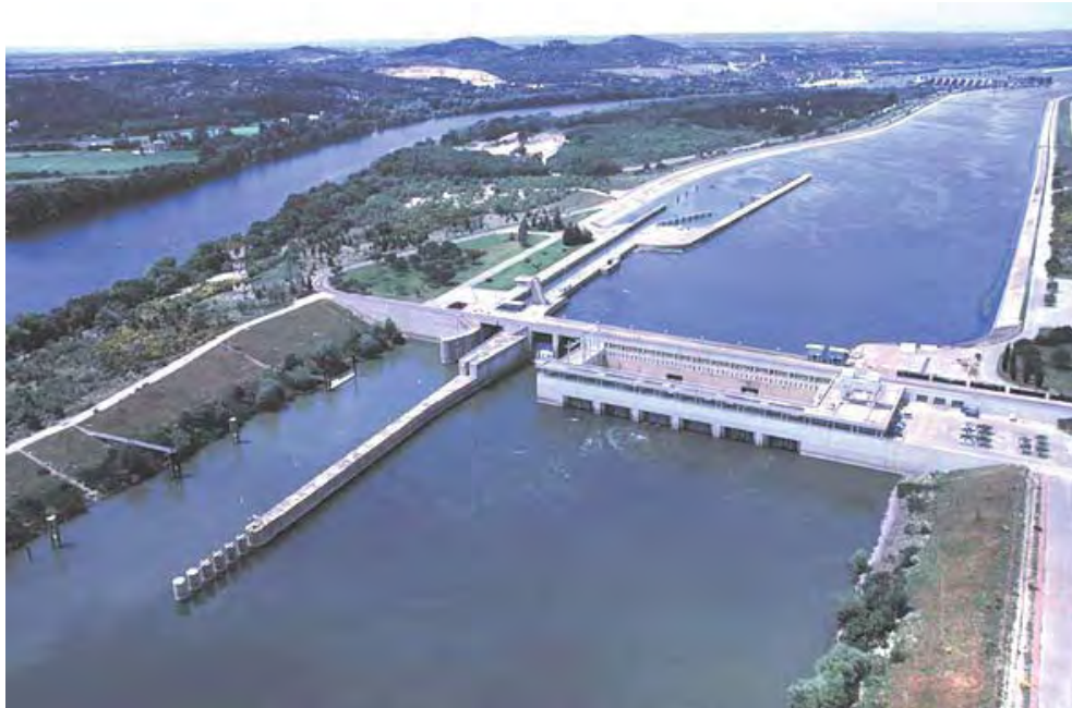
(a) A view of the navigation lock at the Beaucaire power plant on the Rhone River in France.
